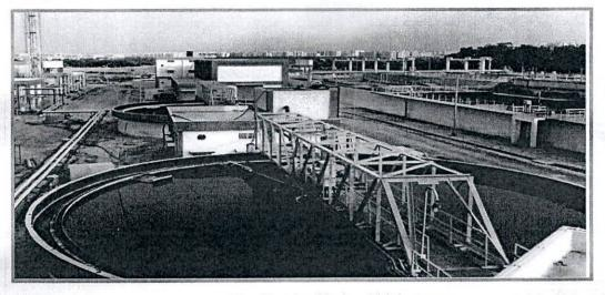
Fig. Gravity Sludge Thickeners
