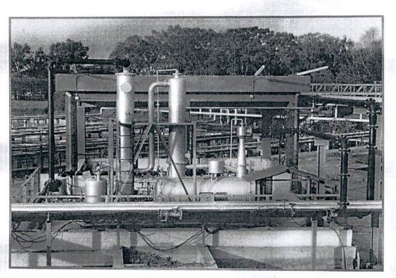
Fig. Biogas Scrubbing System
