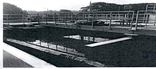
Fig 1: Screenings & Grit Removal System
