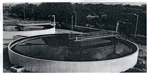
Fig2. Primary Clarifier & Primary Sludge Pumping Station
