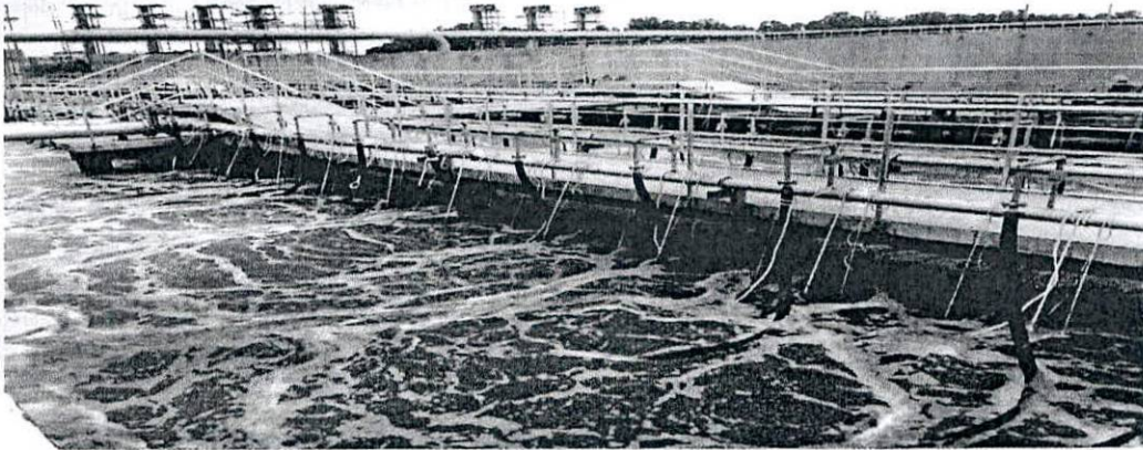
Fig3. Activated Sludge Process with Biological Nutrient Removal
