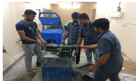
Fig7: Casting of concrete
