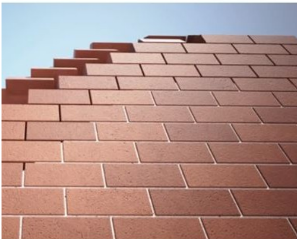
Fig 2. Shows No Plasterwork required
