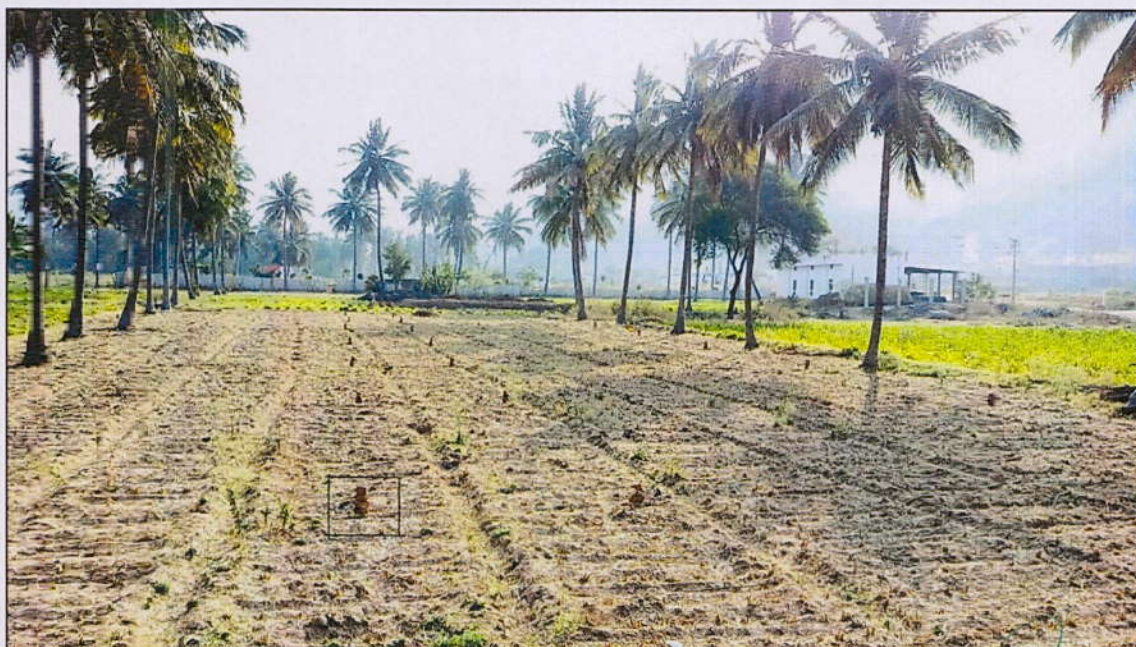
Layout plan Center line alignment with bricks
